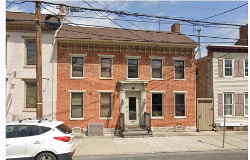
211 Carlisle St, Hanover
