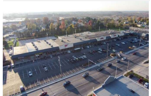
1000 Carlisle St, Hanover
